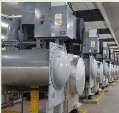
Chillers operating at reduced capacity in T3 due to lower cooling demand
