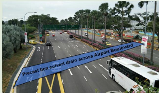
At CAG, besides building the airport on higher platforms above the mean sea level to guard against effects of climate change, the other precaution that we take is to increase the capacity of the airport's drains, to reduce the risk of flooding during intense rain. This is to ensure that Changi Airport continues to operate uninterrupted to serve passengers and customers.
